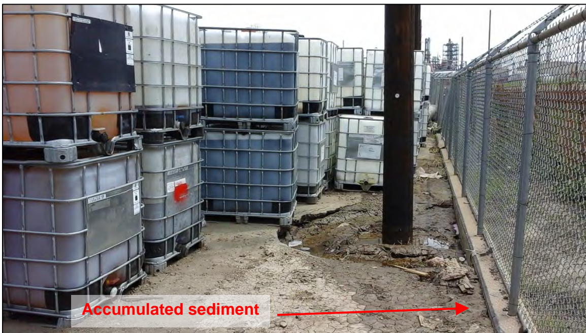
Photograph 26. View, facing north, of sediment accumulation against the Facility's south perimeter wall at the waste chemical and used oil storage area shown in Photograph 25. Note secondary containment was not provided for these totes of waste fluids.
