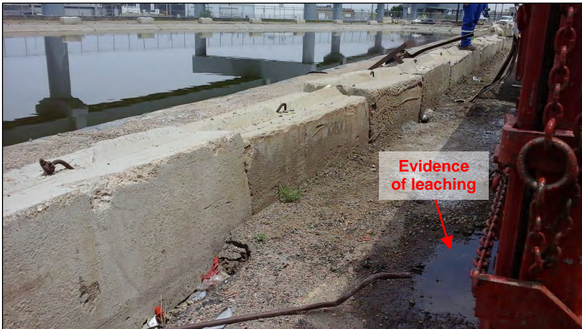
Photograph 35. View of leachate on the ground surface beneath the uncovered scrap and waste dumpsters shown in Photographs 32 and 34.
