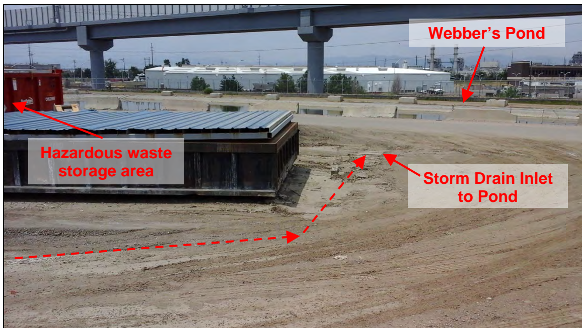
Photograph 39. View of the observed flow pathway from the area with the six (6) red hazardous waste dumpsters to Webber’s Pond, as shown in Photographs 37 and 38. Stormwater runoff from this area enters a storm drain which flows to the adjacent Webber’s Pond.
