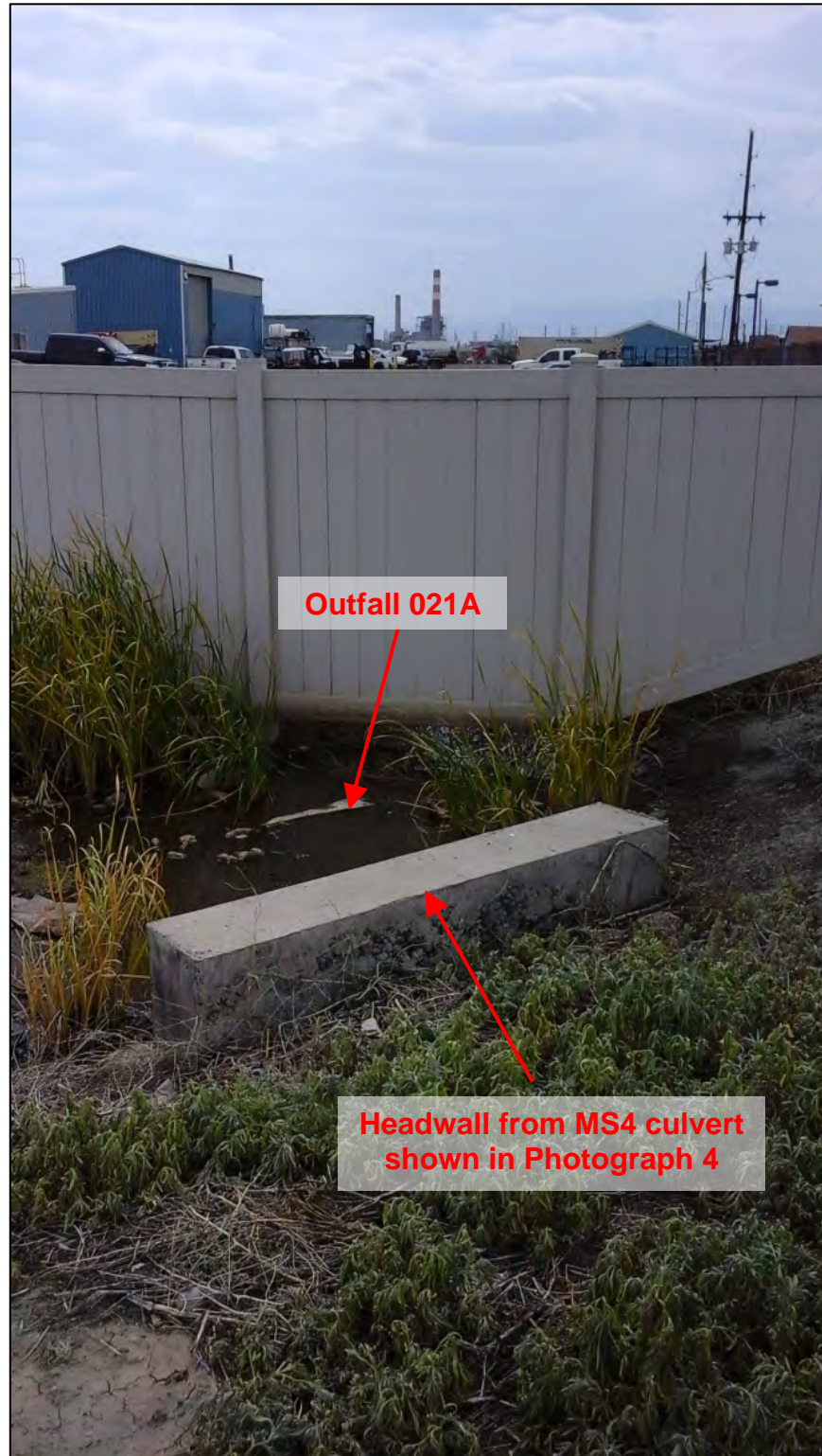
Photograph 3. View, facing west, from the Colorado Boulevard right-of-way, of Outfall 021A at the northeast corner of the Nelson Property. The stormwater detention basin on the northeast side of the property is located behind the white fence. Outfall 021A is noted as the location where accumulated stormwater is monitored and also where stormwater is commingled with stormwater runoff from the City of Commerce City’s MS4 from Colorado Boulevard.
