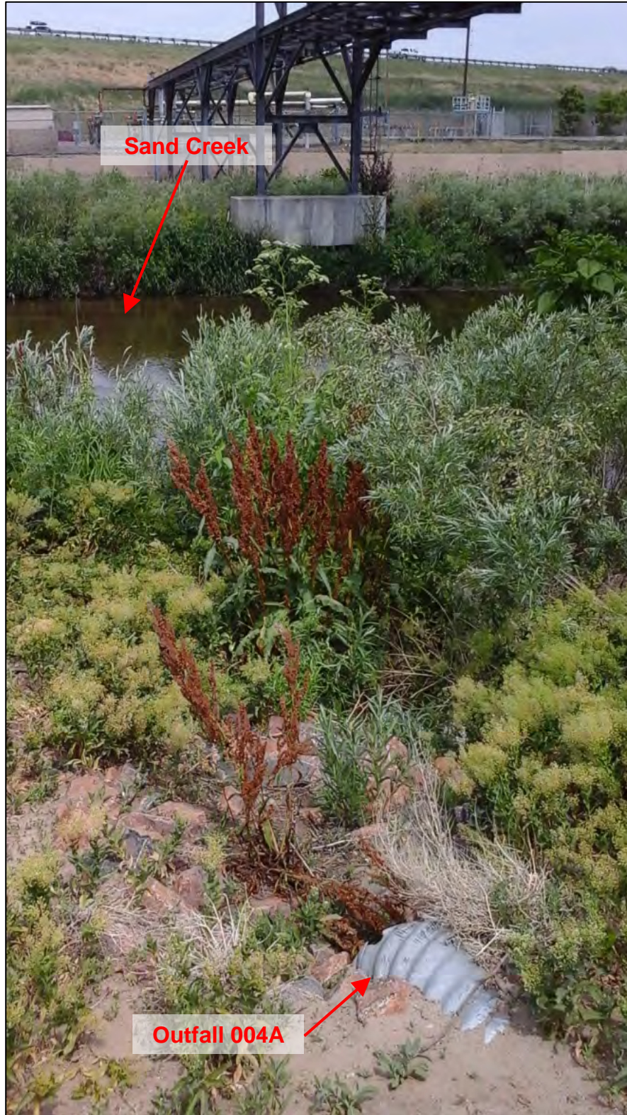
Photograph 2. View of Outfall 004A to Sand Creek from Mary's Pond, shown in Photograph 1.
