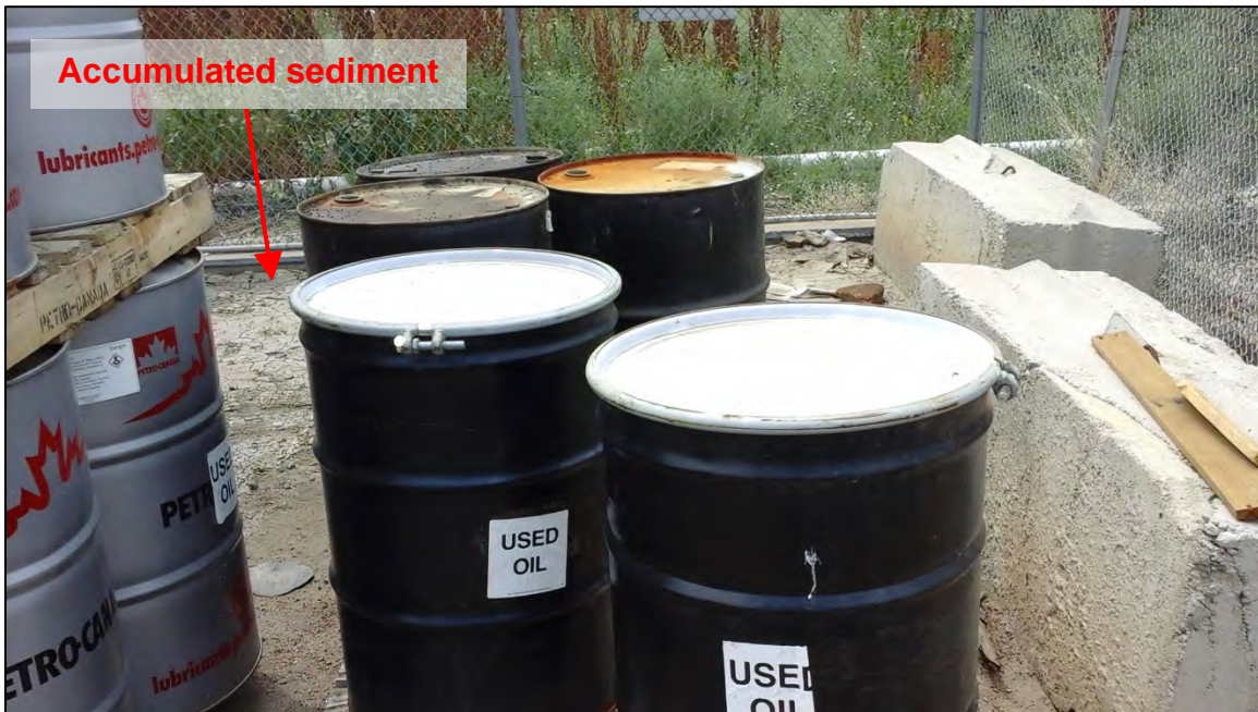
Photograph 28. Additional view of accumulated sediment along the south perimeter wall. Also note secondary containment was not provided for the 55-gallon drums of used oil.
