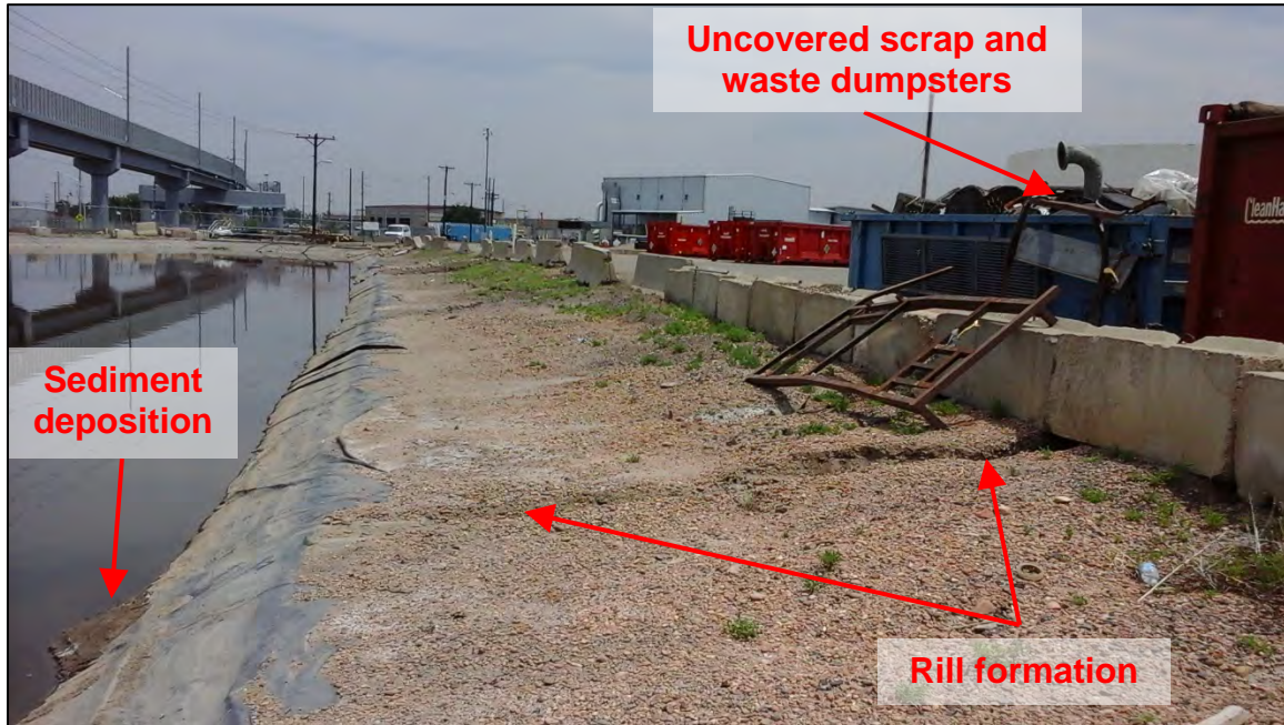
Photograph 32. View, facing north, of rill formation on the east embankment of Webber's Pond. Note the sediment deposited in Webber's Pond below the rill. Also note the uncovered scrap and waste dumpsters located upgradient of Webber's Pond.
