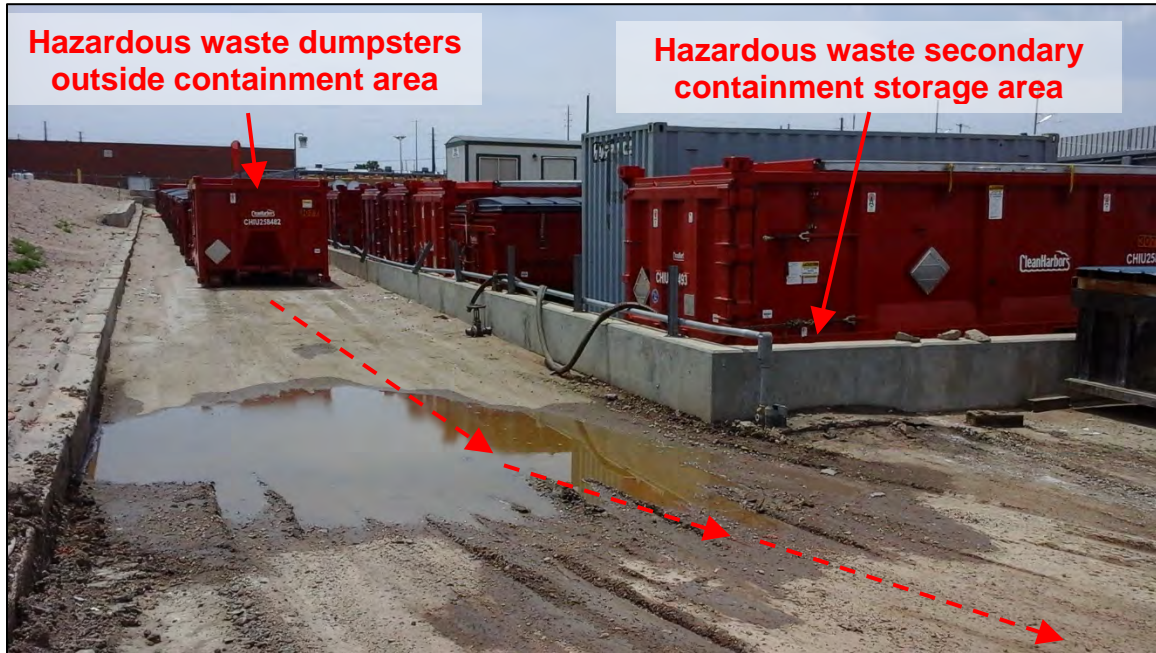
Photograph 38. View, facing south, of the hazardous waste storage area located in Plant 1, east of Webber’s Pond. Red dotted arrow indicates flow direction; refer to Photograph 39 for observed flow pathway to Webber’s Pond.
